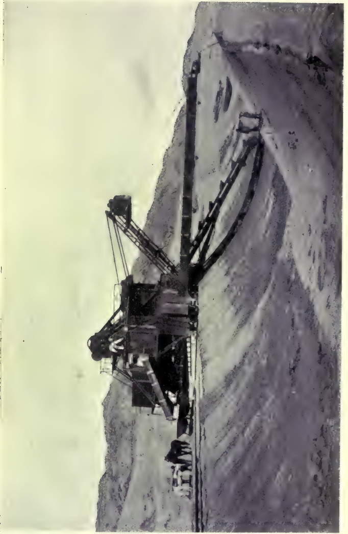
KOLMANSKOP DIAMOND MINES, LTD. DREDGER WITH DRUM SIEVE WORKED BY ELECTRICITY.
